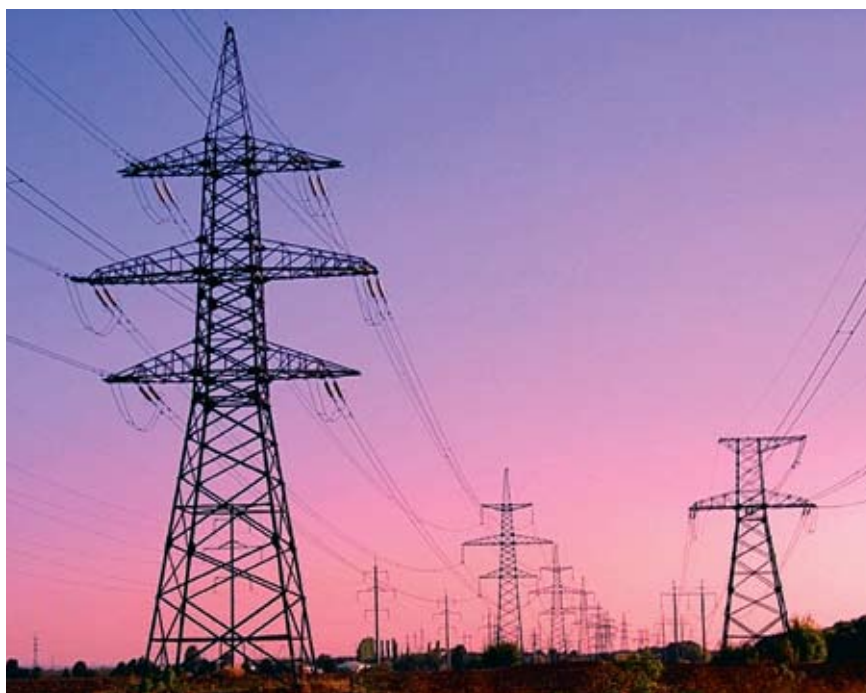
The pipeline ESPO means development of the region also in the power industry
